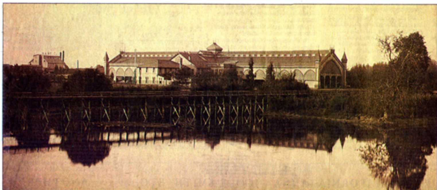
A view of Sacramento's railroad center from across China Slough in a photograph from 1878.
